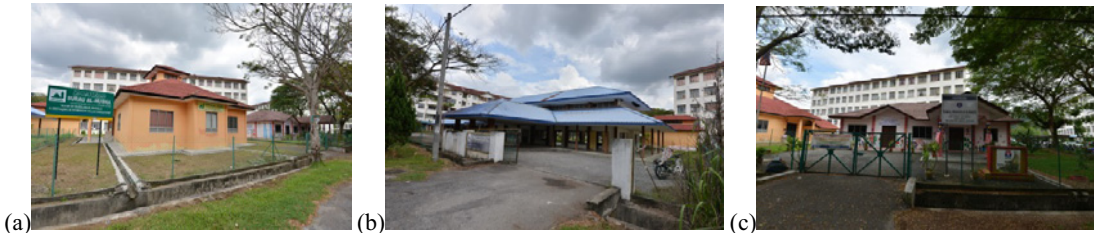
Figure 3: Facilities: (a) muslim prayer hall, (b) multi-purpose hall, (c) kindergarten.
