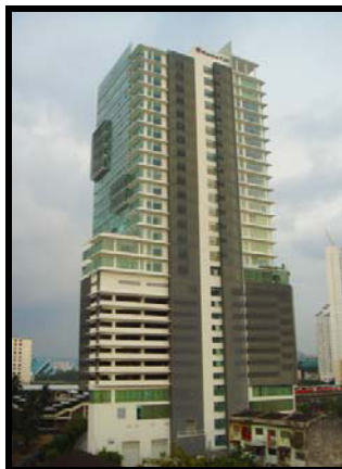
Figure 4: PJD Tower, Kuala Lumpur.
