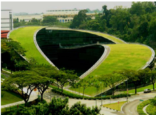
Figure 1: Extensive green roof at School of Art, Design & Media, Nanyang Technological University, Singapore
