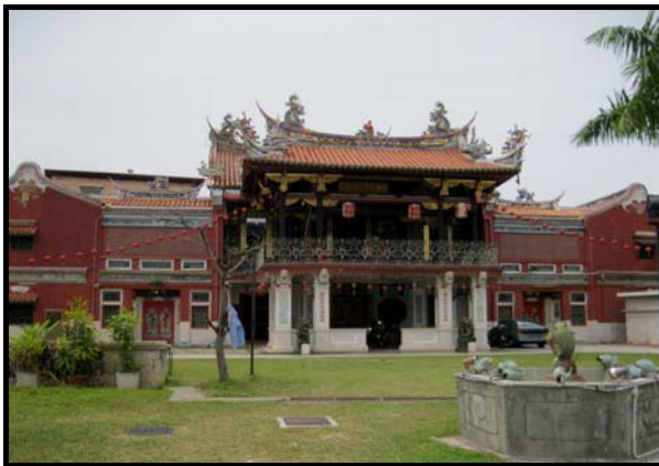
Figure 4: Large open space outside of Cheah Kongsi for mean of escape during fire outbreak.
