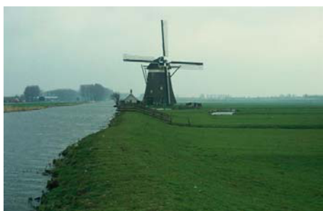
Figure 1. Regional flood defence in the Netherlands (Rijkswaterstaat)
