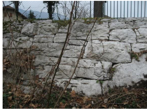
Figure 2. Masonry wall protecting the upstream face of the embankments
