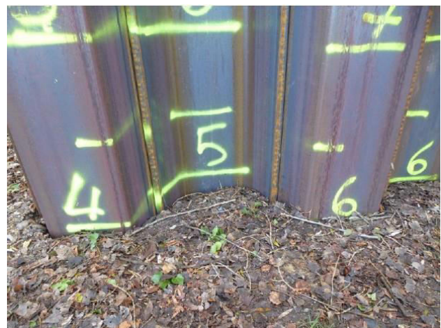
Figure 10. Test of sheet piles driven
