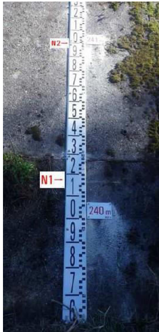
Figure 13. Scale for water level measurements located on the upstream concrete wall
