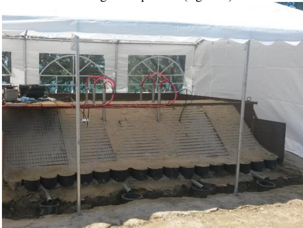
Figure 1. Small experimental embankment
