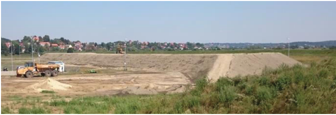
Figure 2. Photography of the experimental levee in Czernichów near Krakow (South Poland)
