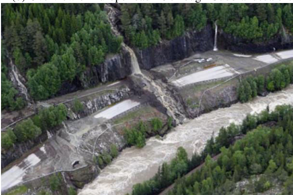
Figure 5. Photos of road damages after the 2011 event. Source: NPRA (2012). Photo: Niklas Eriksson, NPRA.
