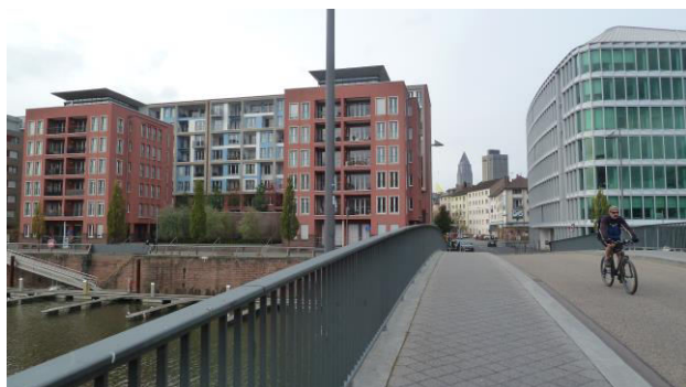
Figure 5. The footbridge linking the Westhafen neighbourhood to the city centre of Frankfurt (CEPRI).
