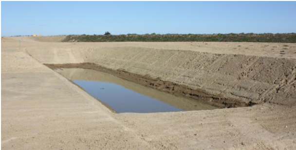
Figure 8 : Stilling basin in February, 2016
