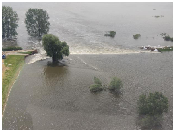
Figure 1. Dike breach on the river Elbe near Fischbeck, June 2013. Photo: Robert Jüpner.
