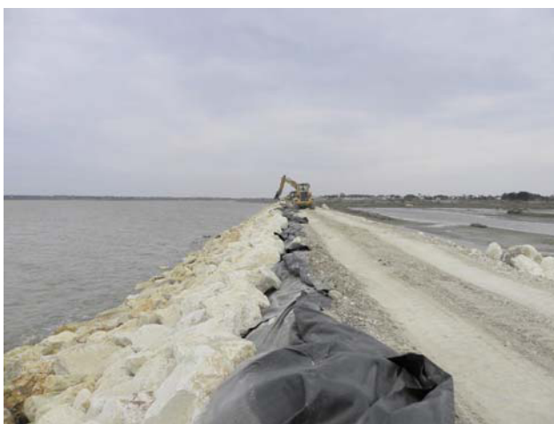
Figure 3: Emergency repair work on a protection dyke
