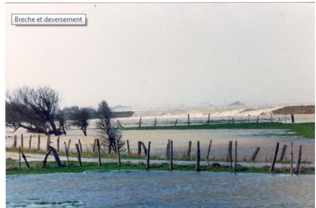
Figure 5: Photography of a breach along the Cayeux coast (storm 1990) Source : Cayeux-citoyens
