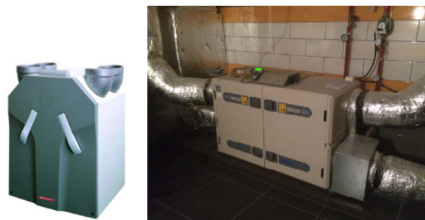
Figure 7. Model of the AERIS 350 LUXE VV recuperator and the same HRU installed in a house (photo by: M. Jarząbek)
