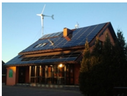
Figure 2. Use of alternative sources of energy: photovoltaic cells and 0.5 kW household wind turbine. “EKOMOTEL na Wierzyńka”. Wieliczka near Krakow (photo by Ł. Steg)
