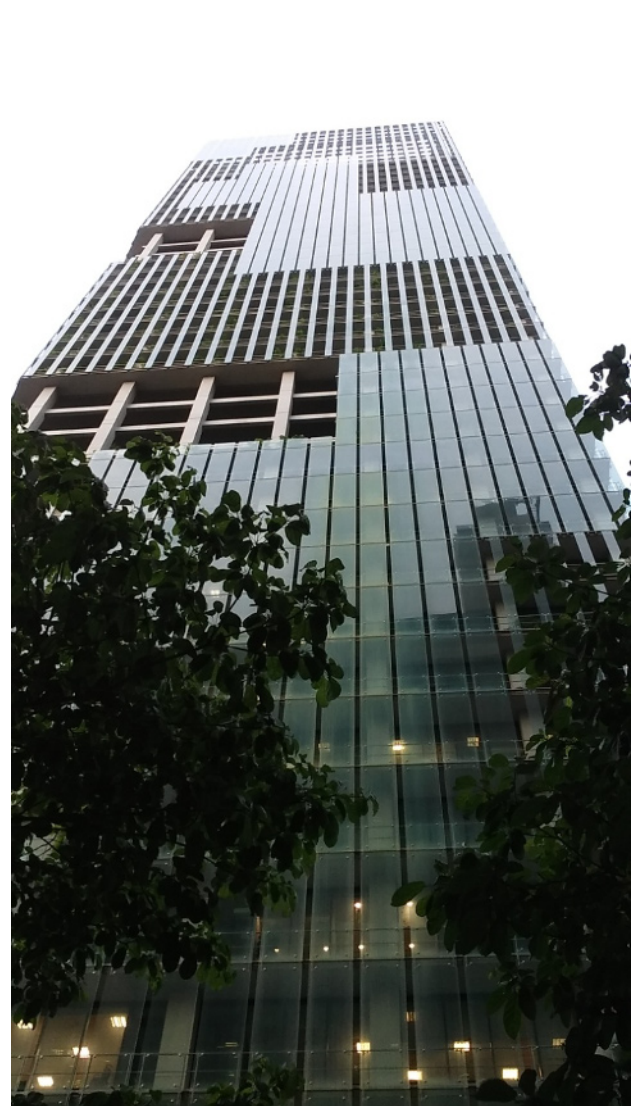
Figure 2. CapitaGreen (2012-2014), Architect Toyo Ito & Associates Architects. Innovatively shaped architecture of the buildings with the introduction of greenery and trees in the entire layout, Singapore (photo by autor, 2016).
