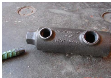
Fig. 5: Half-grouted sleeve connector in US
