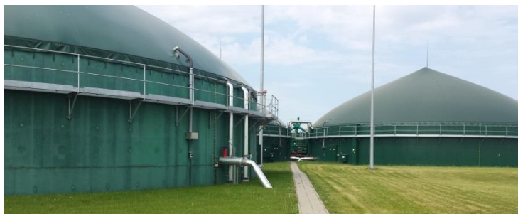
Fig. 1. Large-scale semi-buried digesters located in north-eastern Poland (photo of the author).
