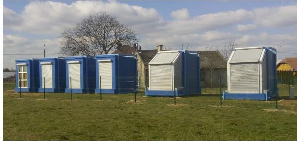
Fig. 1. View of the research chambers at the Rzeszów University of Technology.
