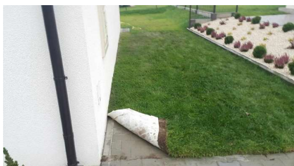
Fig. 7. Removed artificial surface - paving stones and parking space after receiving the object. Source: own study.
