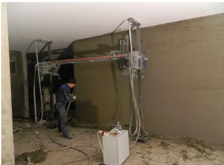
Fig. 1. Plasterer robot PlasteRUS Foreman.
