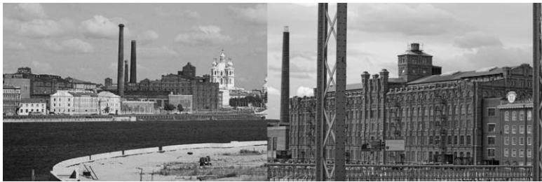
Fig. 5. Panorama of Nevskaya Paper Mill and Second weaving mill building.
