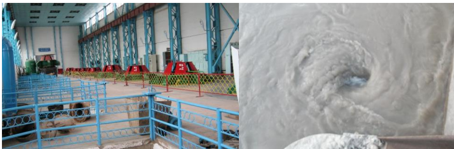
Fig. 1. Whirlpool funnels in the intake and machine room pumping station Amu-Zang 2
