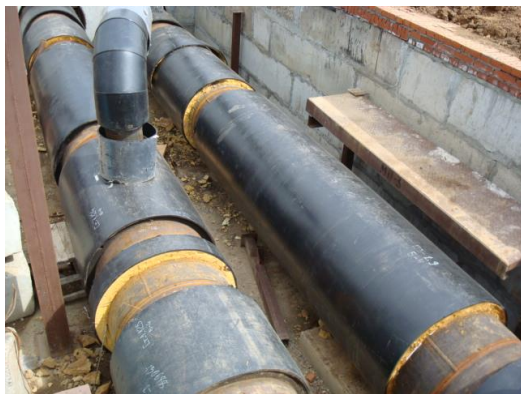
Fig. 4. The use of cutting pieces of pipe on one of the pipelines.
