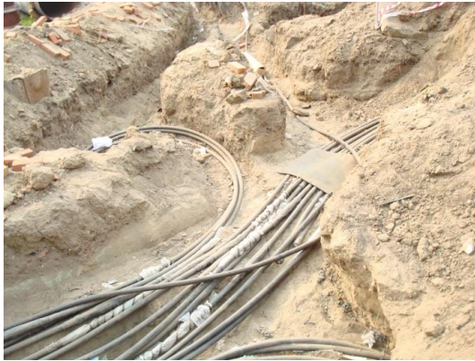
Fig. 3. Detected power cables not marked on topographic survey.
