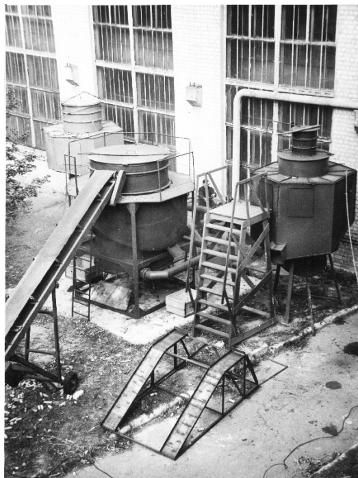
Fig. 6. Block of installations for threshing at Kharkov Aviation Institute, tubes with a diameter of 1.2-2 m.
