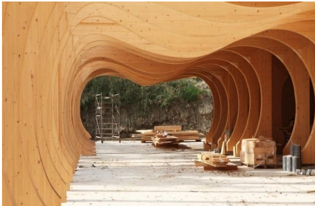
Fig. 2. Installation of glued laminated frames during the construction process. (Source: https://www.archdaily.com/775276/nido-dinfanzia-a-guastalla-mario-cucinella-architects?ad_name=single-scroll )
