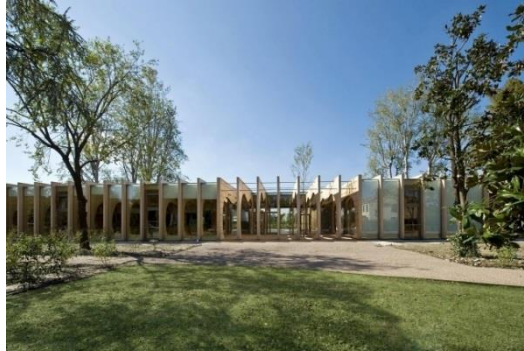
Fig. 1. Exterior of a preschool in the town of Guastalla. (Source: https://www.archdaily.com/775276/nido-dinfanzia-a-guastalla-mario-cucinella-architects?ad_name=single-scroll )
