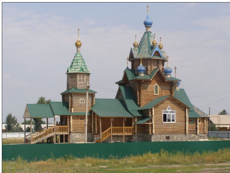
Fig. 8. Church of the Mantle of our Lady, Yuzhnouralsk town. Built in 2008. Architect N.S. Akchurina. Photograph by E.V. Ponomarenko
