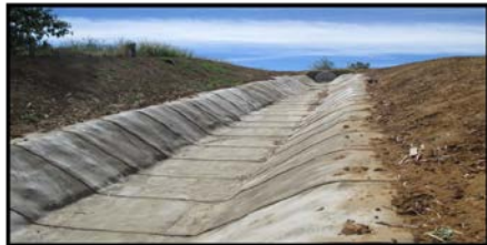
Fig. 2.1. – Concrete canvas-lined irrigation canal.
