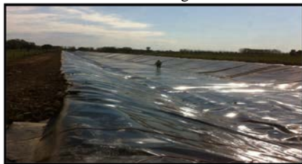
Fig. 2.2. – Geosynthetic membrane-lined irrigation canal.
