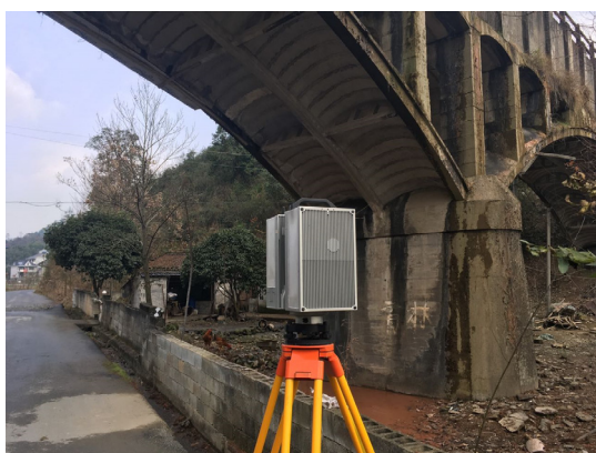
Fig. 1. 3D laser scanning for the aqueduct body
