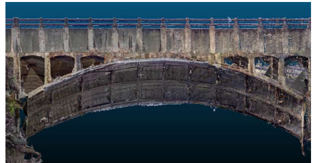
Fig. 2. 3D point cloud of first span aqueduct
