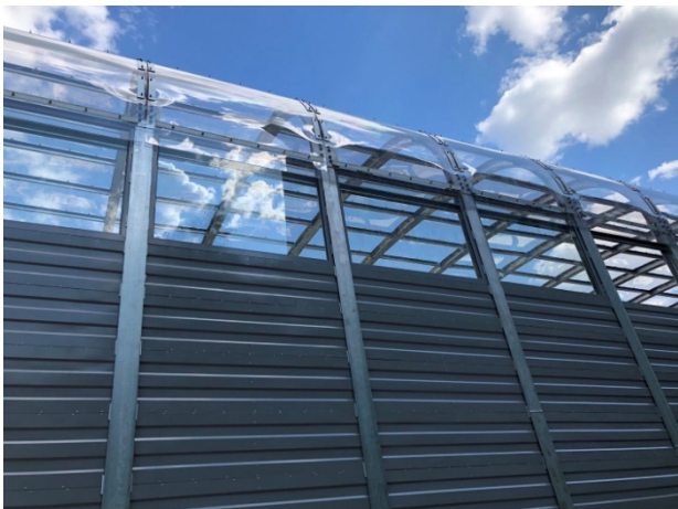
Fig. 9. Actual Picture of Ground Subgrade Noise Barrier After Installation
