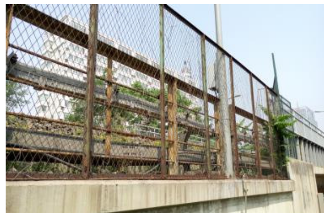
Fig. 5. Status Quo of Ground Subgrade - Blocking Net
