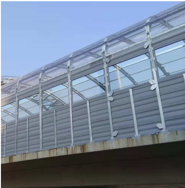
Fig. 8. Actual Picture of Viaduct Noise Barrier After Installation
