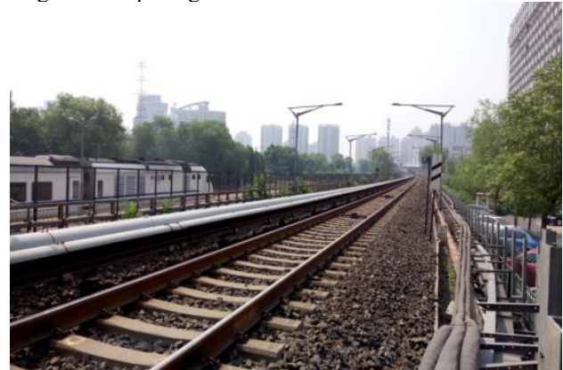
Fig. 4. Status Quo of Ground Subgrade
