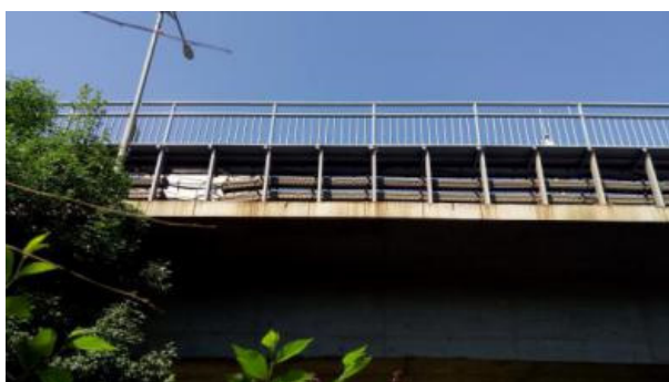
Fig. 3. Status Quo of Viaduct - Section without Noise Barrier
