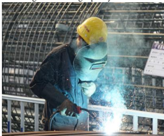
Figure 12. Rebar processing plant, prefabricated plant, tunnel steel structure using carbon dioxide protection welding
