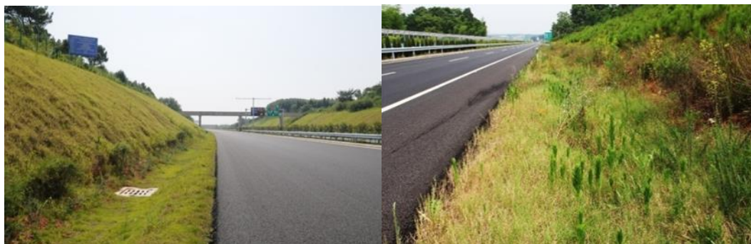
Figure 2. Photo of ecological side trench system technology application case
