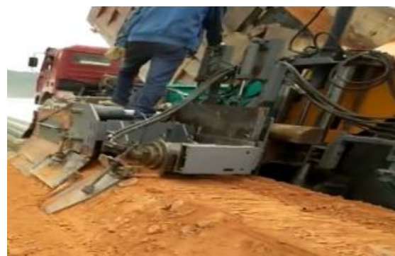
Figure 12. Spreading technology of earth shoulder
