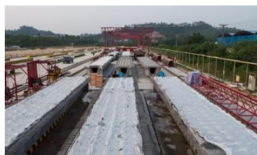
Figure 3. Main line subgrade as precast beam yard
