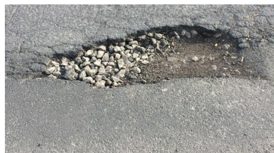
Fig4. Material recovery from the bituminous layer
