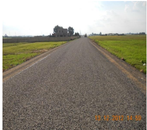
Fig.2. Photo of the section at the end of works
