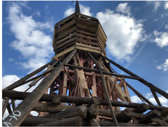
Fig. 10. The structure of the drum, bulb and spire. The author of the photographs is Zhivotov D. A.
