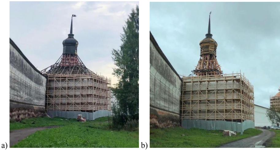
Fig. 14. a) - dismantling of the crate, b) - disassembly of the crib. The author of the photographs Galaktionova O. S.
