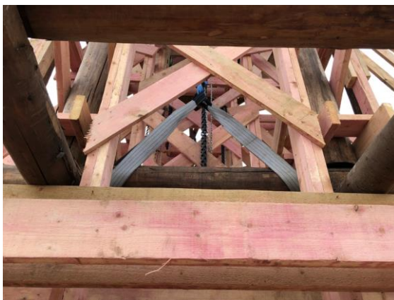
Fig. 11. Arrangement of 8 hoists for lifting the roof of the tower. The author of the photographs is Zhivotov D. A.
