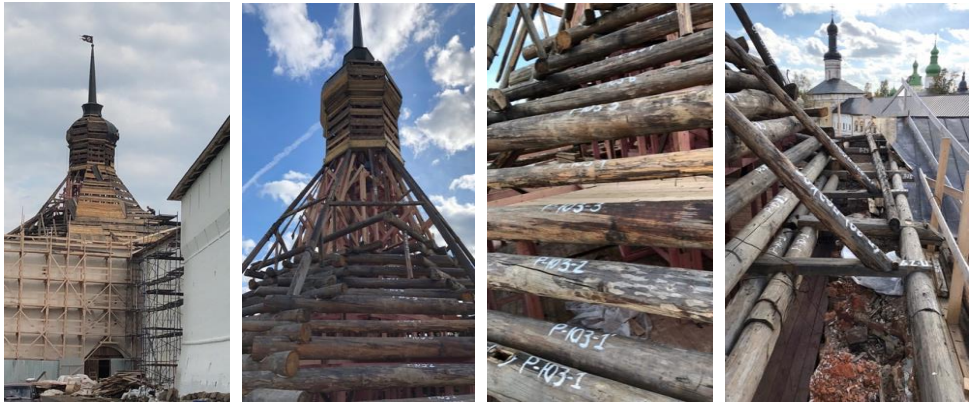
Fig. 8. Marking of wooden elements of the roof. The author of the photographs Galaktionova O. S.
