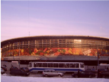
Fig. 2. Baumansky market before collapse, Moscow, Russia.
