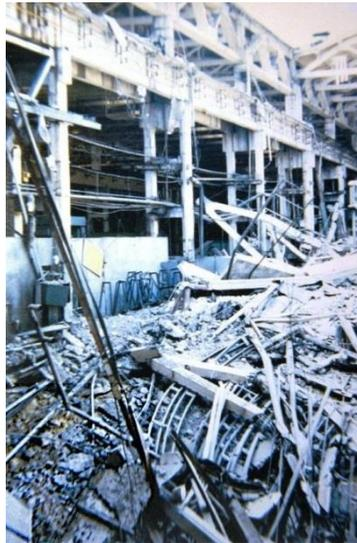
**Fig. 7.** The edge of the sagging-collapse sinkhole and the result of caused by its formation partially destruction of an industrial building (Dzerzhinsk, Nizhny Novgorod Region, 1992).
