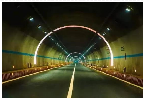
Figure 2. Application of tunnel energy storage luminous reflector
