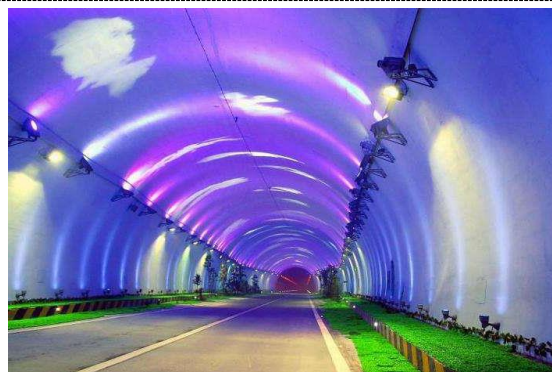
Figure 1. Application of landscape lighting belt in tunnel
