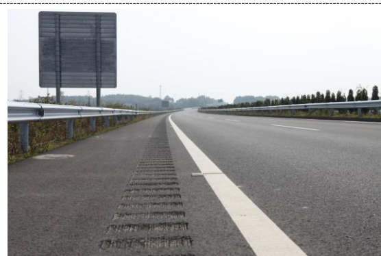
Figure 4. Roadside vibration band application
