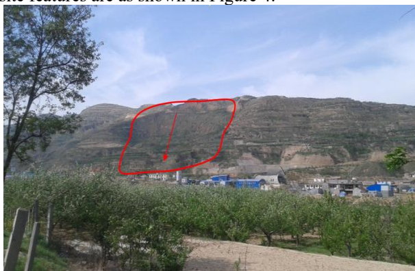
Figure 4 Country tunnel morphology at the scene
