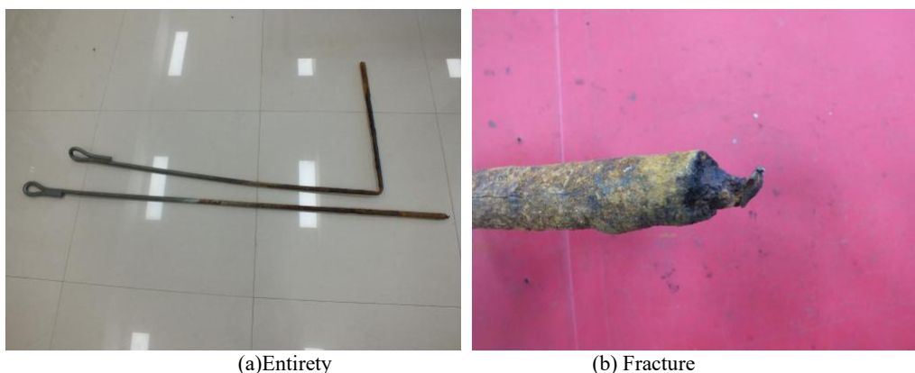
Figure 1 The macro morphology of the corroded guyed rod.
