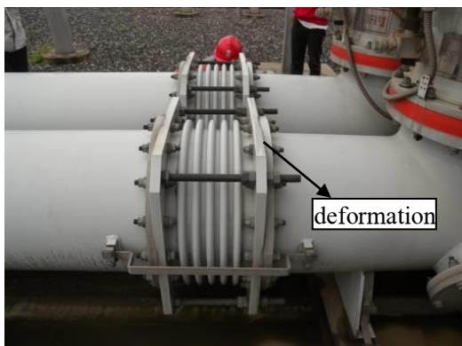
Fig. 1. Morphology of flange deformation.
