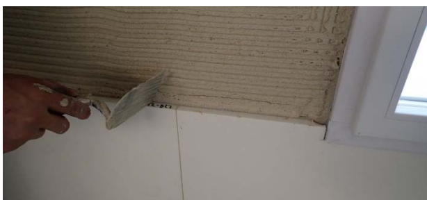
Fig. 8. Avoiding adhesive from entering in joints between insulation panels.
