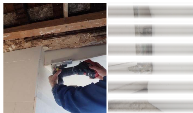
Fig. 10. Modelling the insulation panel around details such as connection to historic wood beam ceiling, window hinge / Luxembourg.
