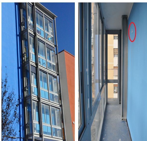
Fig. 2. On the left, general view of the sunspaces on the South façade of the studied building; on the right, internal view of the studied sunspace with the recording thermometer marked.
