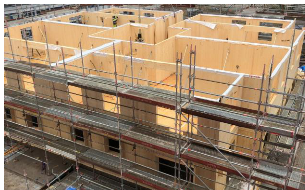
Fig. 1. Ongoing assembly of CLT frame without weather protection in central Sweden.
