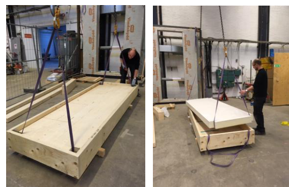
Fig. 3. The assembly of the mock-up.
