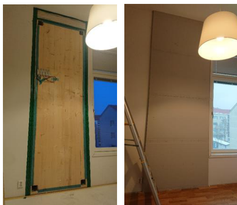
Fig. 5. The completion of the mock-up installation.
