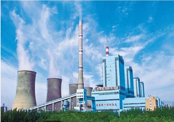
Fig. 1. Power Plant in Shentu.
