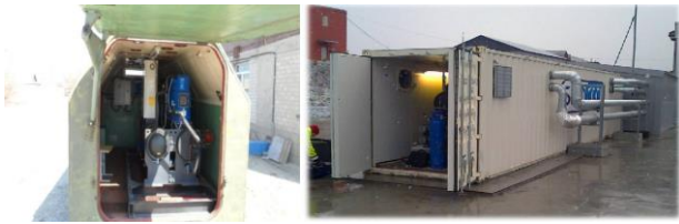
Fig. 3. General assembly of modular heat pump (MHP).
