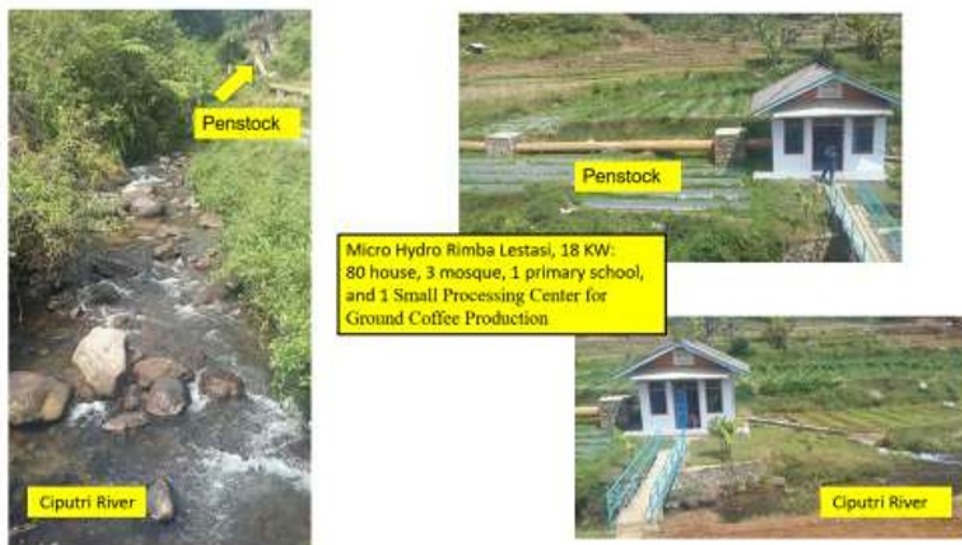
Fig1. Micro-Hydro Rimba Lestasi, 18 KW in Tangsi Jaya, Bandung
