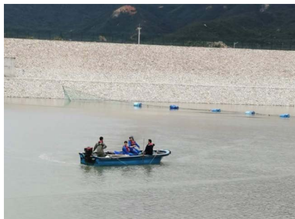
Fig.2 Acoustic survey of seawater storage in Taishan nuclear power plant
