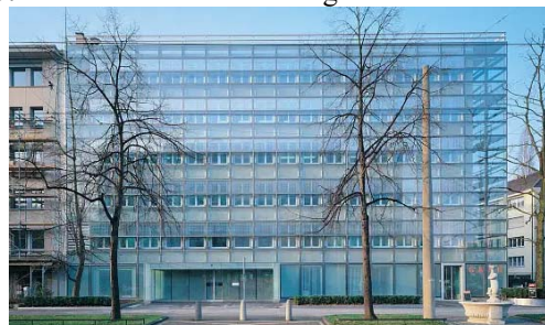
Fig.4. The SUVA office building after renovation
