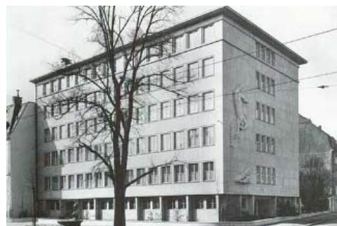
Fig.3. The SUVA office building before renovation
