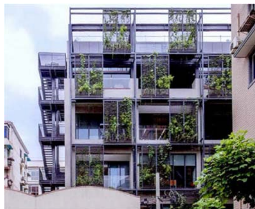
Fig.6. Facade of the renovated Shendu Building
